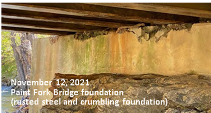
View of Paint Fork Bridge structural concerns
