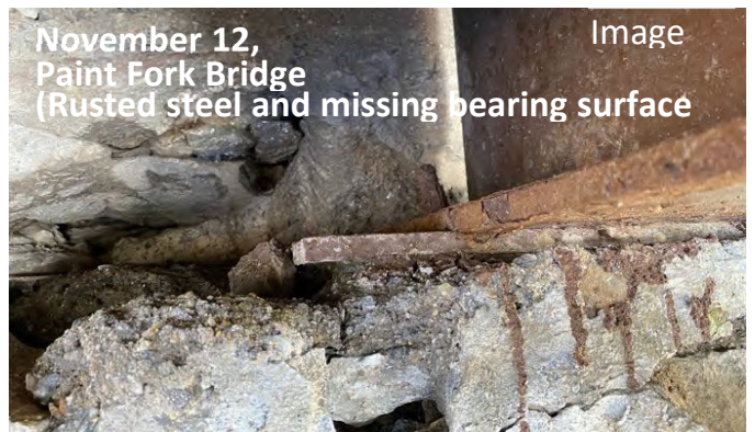
View of Paint Fork Bridge structural concerns
