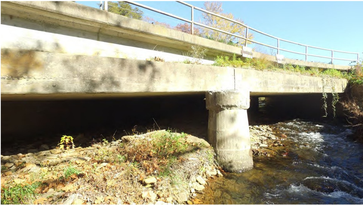
Barnardsville Highway (NC197) culvert crossing of North Ivy Creek looking upstream
