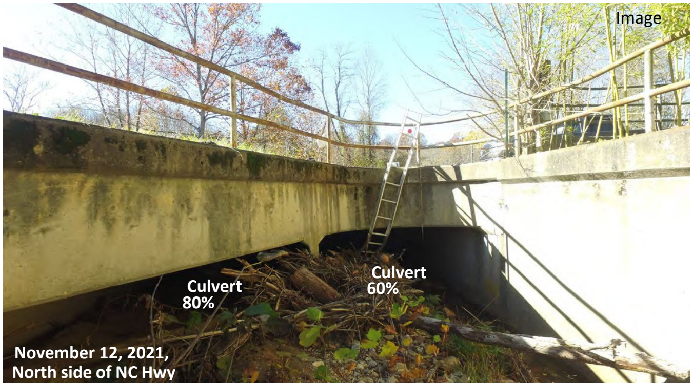
Barnardsville Highway (NC197) culvert crossing of North Ivy Creek looking downstream
